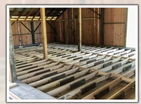
Completed underfloor framing for North end.
