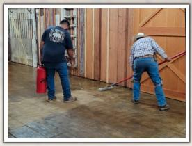
Staining the stamped concrete floor.
